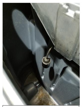
The float switch is several inches below the top of the recovery tank
