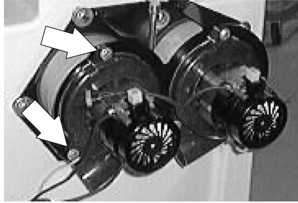
5. Remove the vacuum fan from the bracket.
