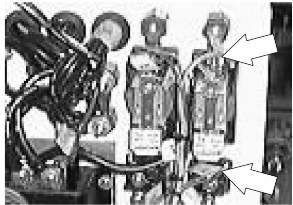
6. Remove the two hex screws holding the 36V relay to the control panel. Remove the relay from the machine.
