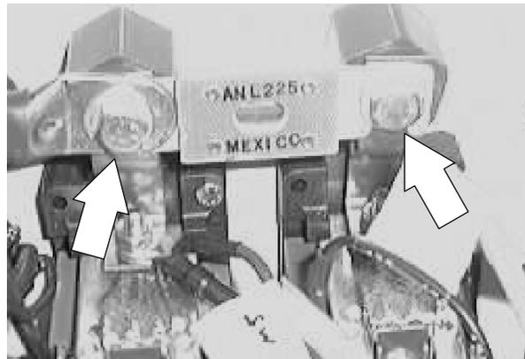
6. Pull one end of the fuse up, then remove the fuse from the standoff.
